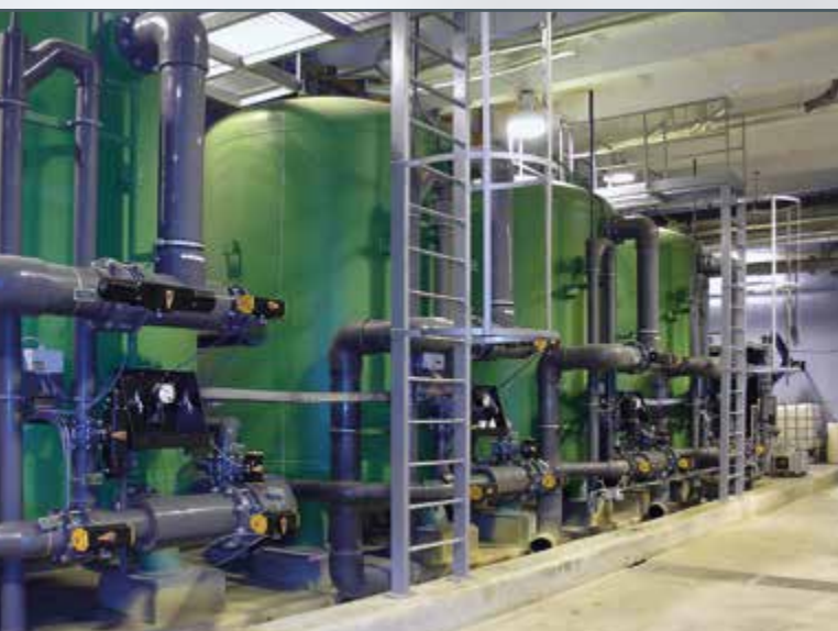
Continuous-flow adsorber in a water treatment plant
