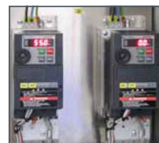
Frequency converters for controlling the pumps
