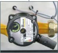
Energy-efficient circulating pump with adjustable differential pressure control (efficiency class A)
