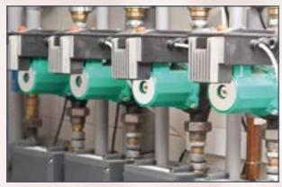
High-efficiency heating circulating pumps provide the same capacity as conventional pumps while consuming up to 80% less power
