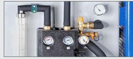
The solar circuit station contains a circulating pump and key components for safe operation.
