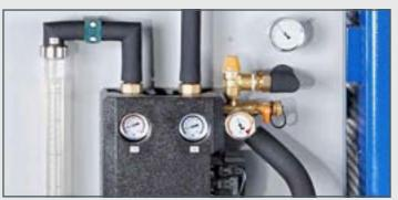
The solar circuit station contains a circulating pump and key components for safe operation.
